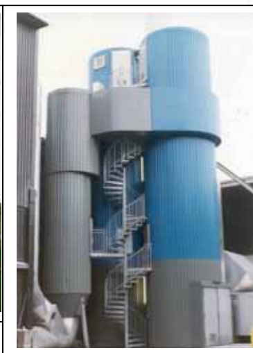
Aluminum Smelting Furnace
